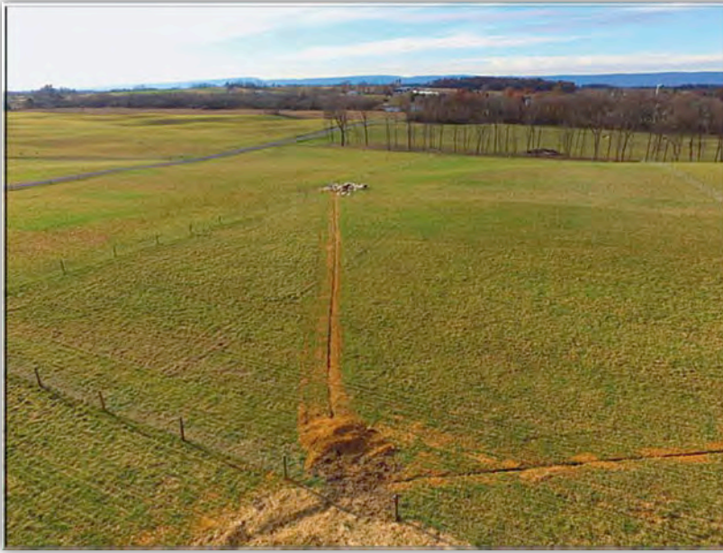
Drone photo of water & electric lines. I document underground work for later reference.
